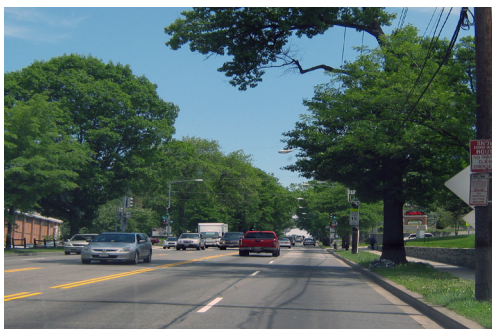
Driving east on the project route.
